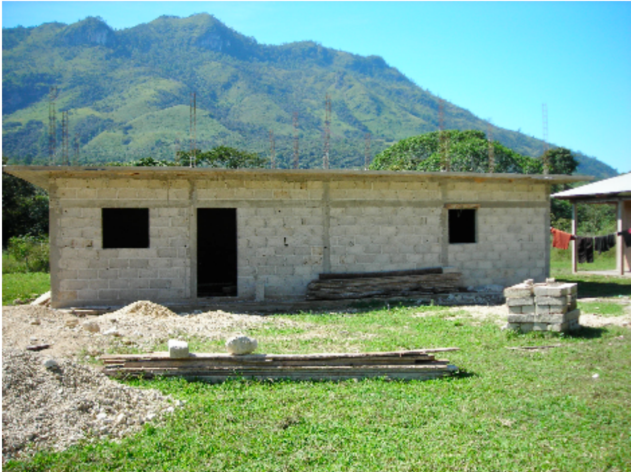
Pharmacy Warehouse under construction.
